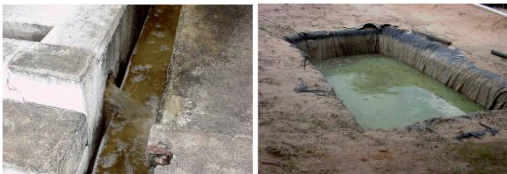
Figure 5. Deposition of residue washing waters.
